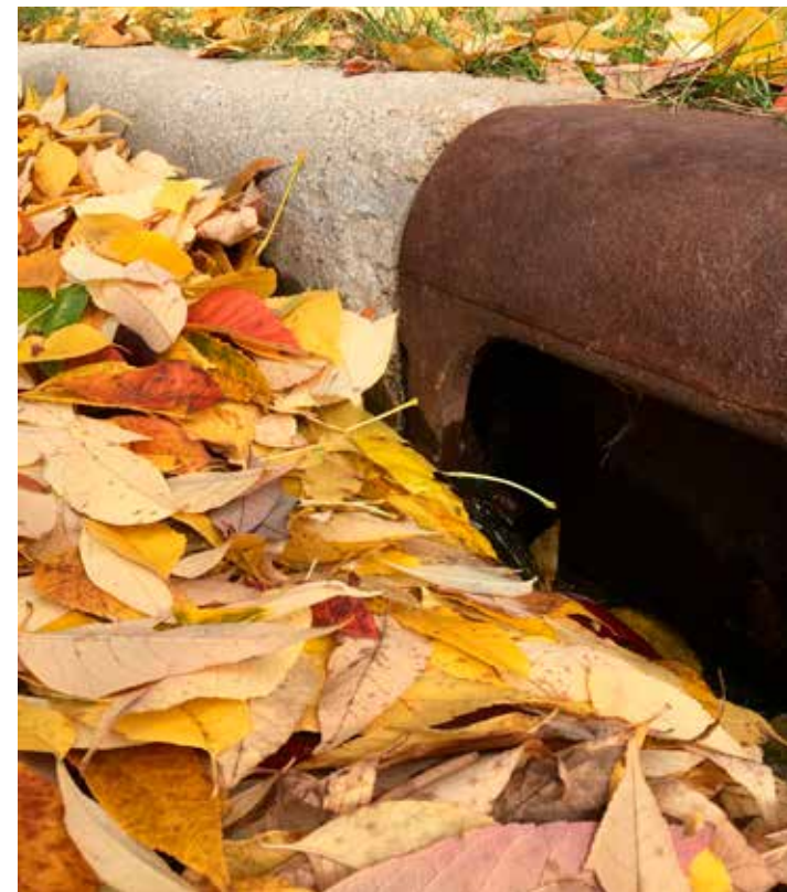
The USGS Madison, Wisconsin study found that stormwater nutrient levels were highest during the fall months when the amount of organic debris on streets was at its peak. Photo by Bill Selbig
