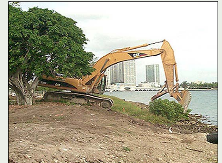
Initial slope grading at Parrot Jungle Island. Photo by Jeff Shimonski
