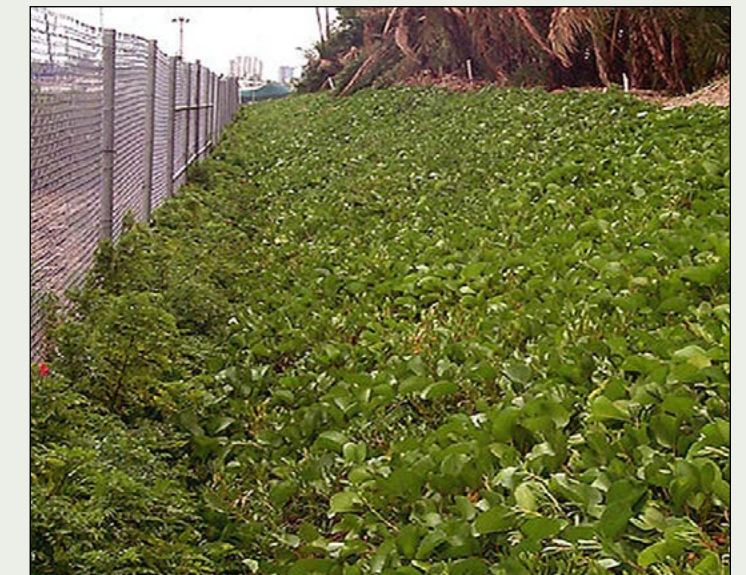
Five months after planting, carefully selected vegetation was doing its job nicely for the perimeter of Parrot Jungle Island. Heavy rainfall never washed out these planted slopes. Photo by Jeff Shimonski
