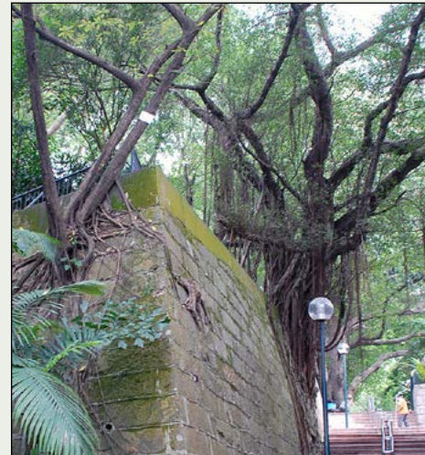
In Hong Kong, one sees the famous stone retaining walls with the ever-attendant Chinese banyan trees growing on top of them. Photo by Jeff Shimonski
