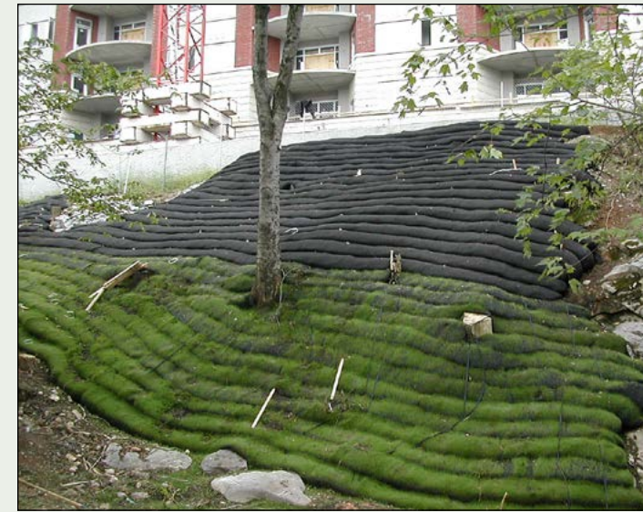
The Chattanooga slope in mid-project. Photo by Gene Hyde
