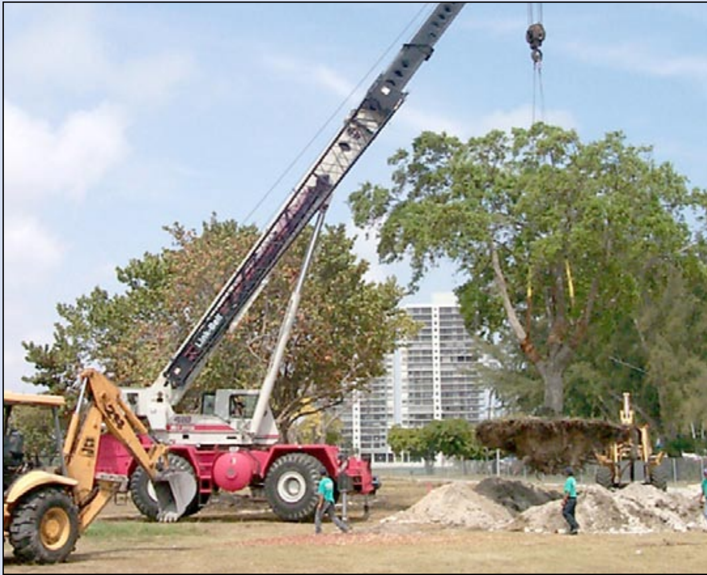
A 60-ton, all-terrain crane was used to move this live oak ( Quercus virginiana ), in the first of two moves ten years ago in Miami. This tree and another similar sized live oak have doubled in trunk width since relocation. Photo by Jeff Shimonski
