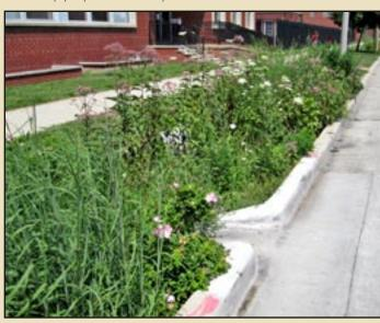
In Milwaukee, Wisconsin, runoff from the roadway enters the bioswales through curb cuts and filtrates through two layers of engineered soil and crushed stone. Photo by Scott Baran
