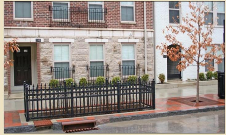
Street-side bioretention wells in Upper Arlington, Ohio capture stormwater from the street before the water enters the storm sewer system. Carefully selected shrubs and perennials fill the well adjacent to sawtooth oak (Quercus acutissima). Photo by Steve Cothrel
