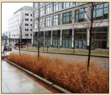
Red maples (Acer rubrum) and grasses fill rain garden structures that allow stormwater to enter both through openings in the street curb and scuppers in the stone edge along the sidewalk. Photo by Steve Cothrel
